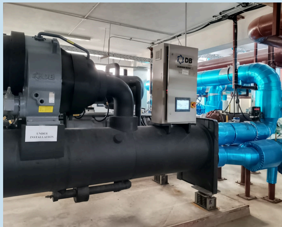
Centrifugal Chiller (USA), 02-Nos & Cooling Tower, 03- Nos, Hormone Building
